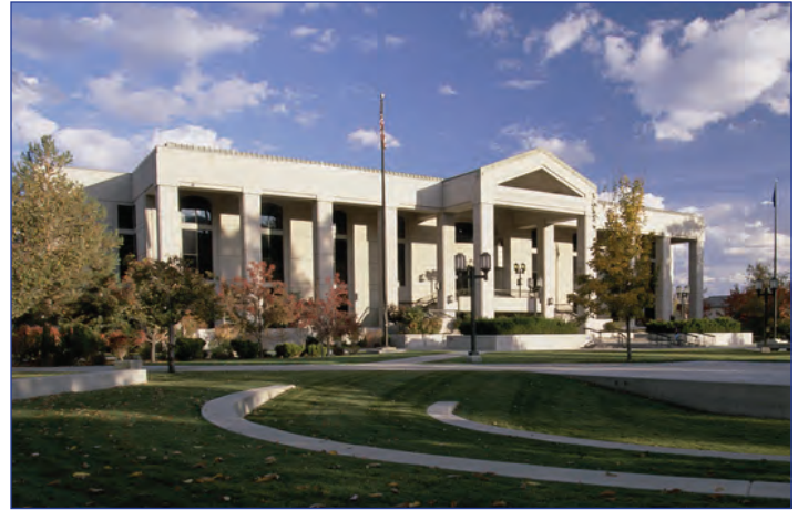
The Nevada Supreme Court Building
